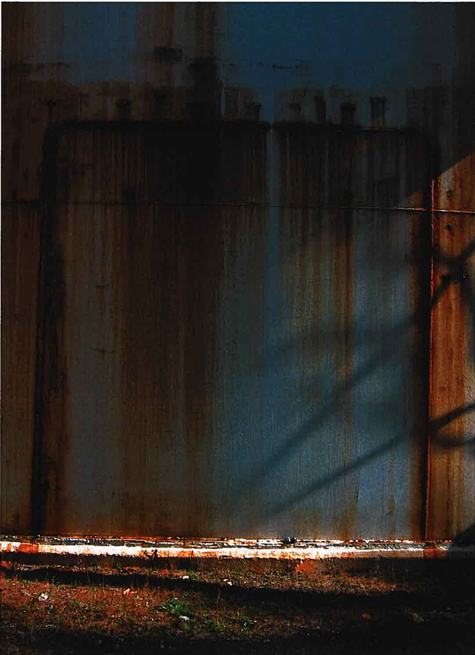
12. Corrosion on shell and door sheet.
