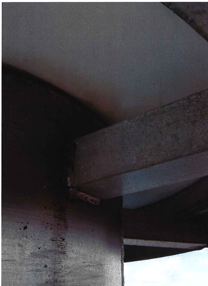
37. Underside of clog-resistant vent.
