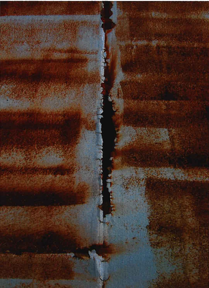
32. Peeled coating and corrosion on roof.
