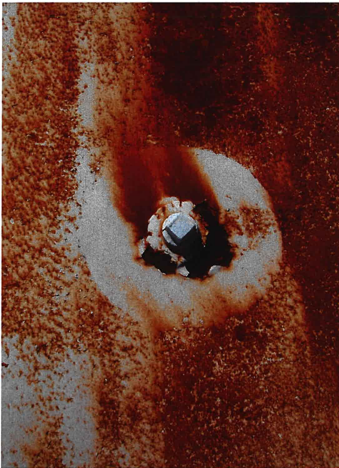
35. Threaded and plugged coupling.
