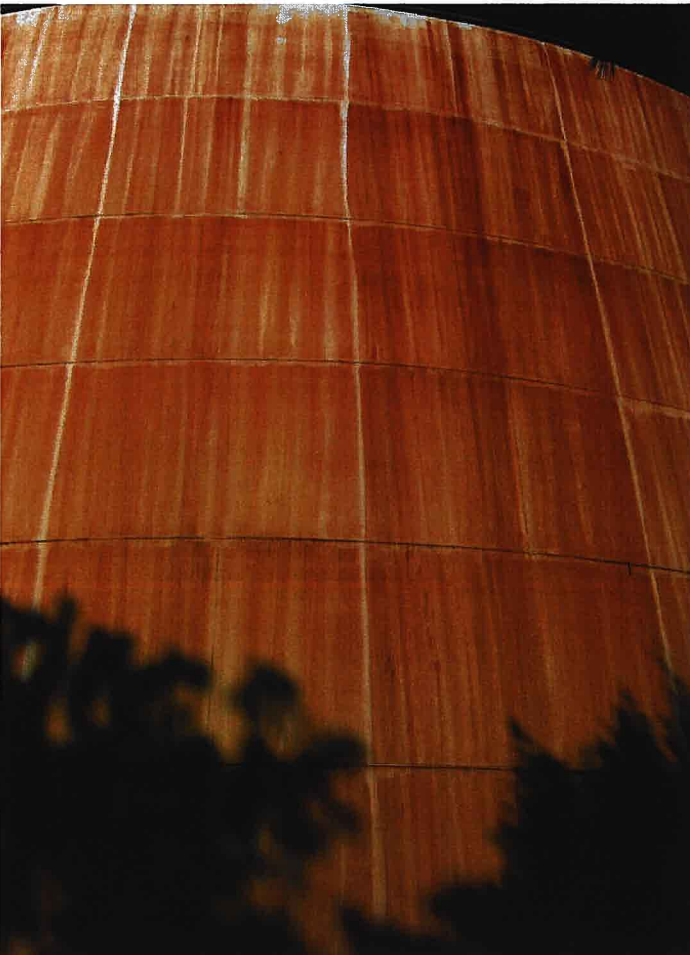
14. Rust staining on shell.
