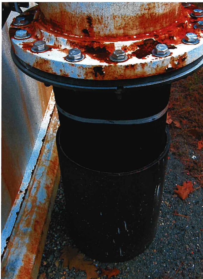
18. Overflow pipe, elastomeric check valve, and discharge pipe.
