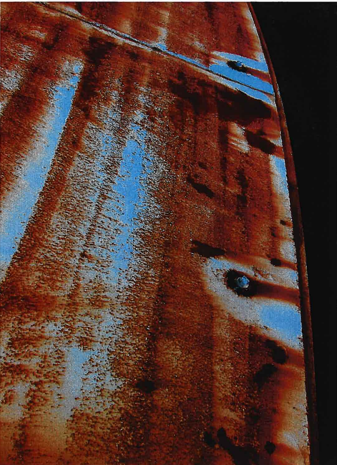
34. Threaded and plugged couplings, and corrosion on roof.
