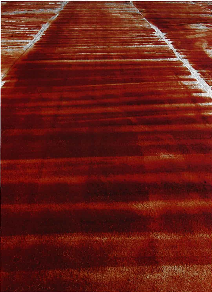
33. Corrosion on roof.
