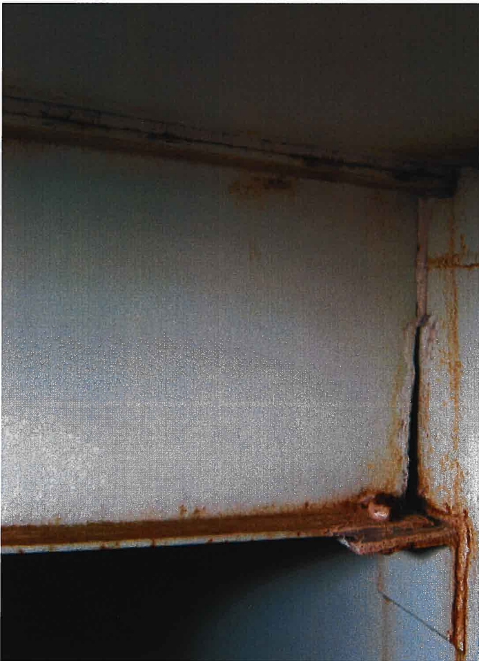
46. Rafter attachment to shell.
