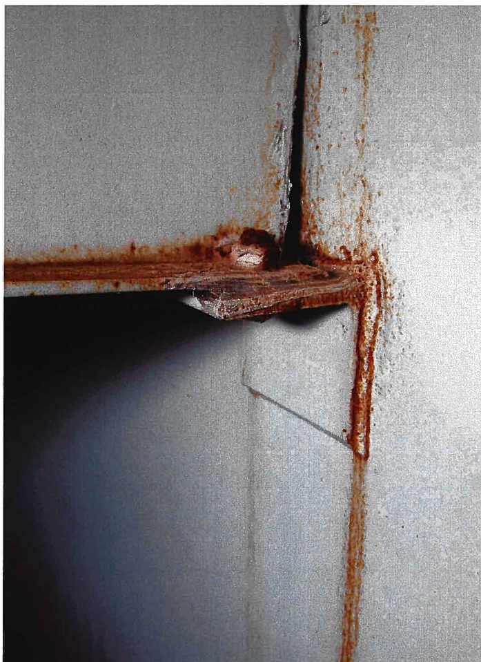
47. Corrosion and rust staining on attachment clip and bolt.
