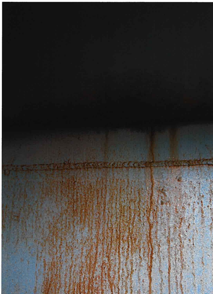
48. Corrosion and rust staining along roof-to-shell connection.
