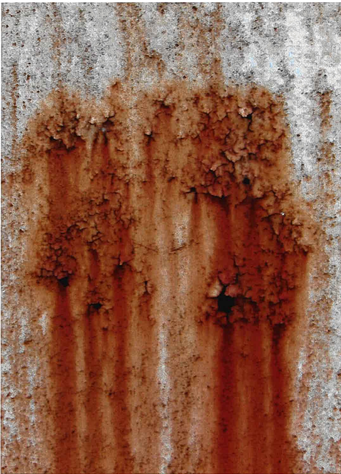
13. Peeled and cracked coating and corrosion on shell.
