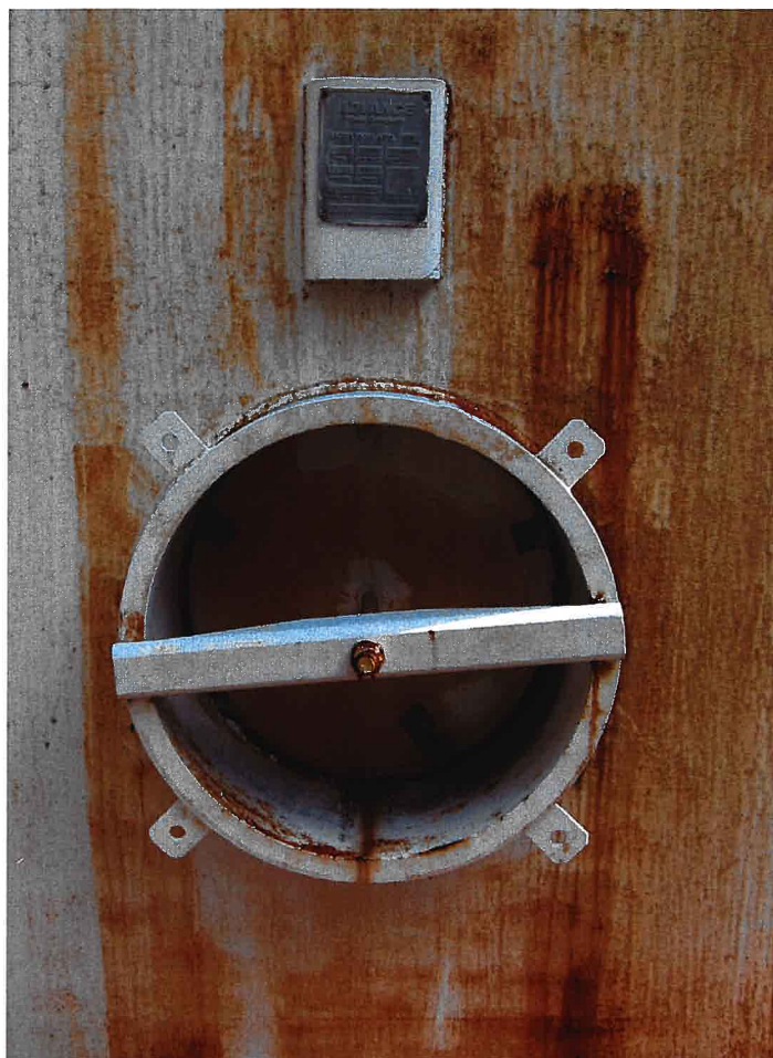
15. Shell manhole and tank nameplate.
