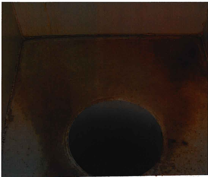
50. Overflow inlet weir box.
