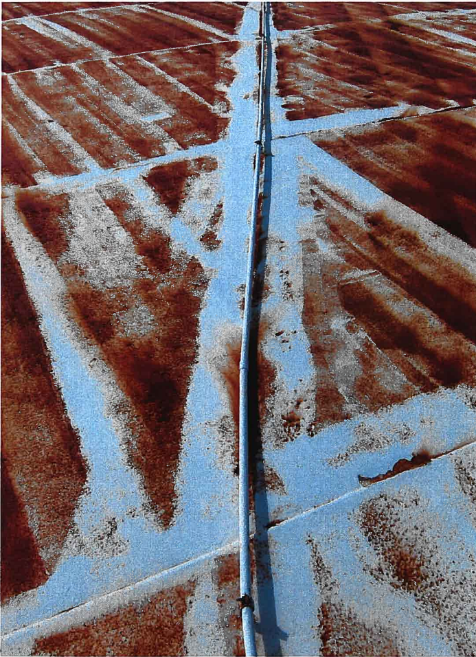
31. Corrosion and conduit on roof.
