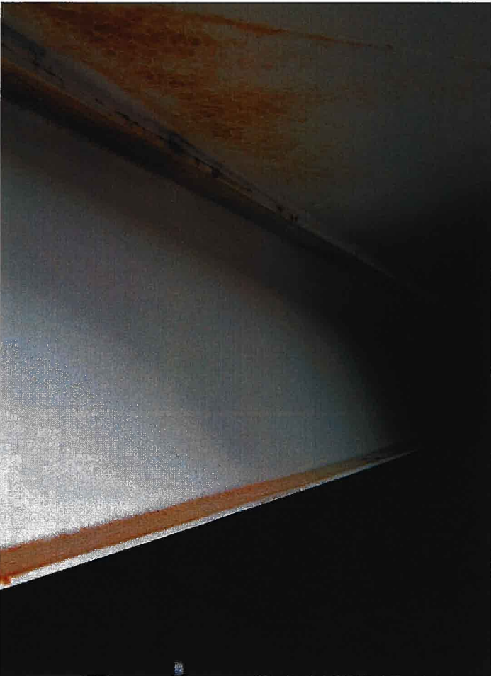
42. Rust staining along rafter.
